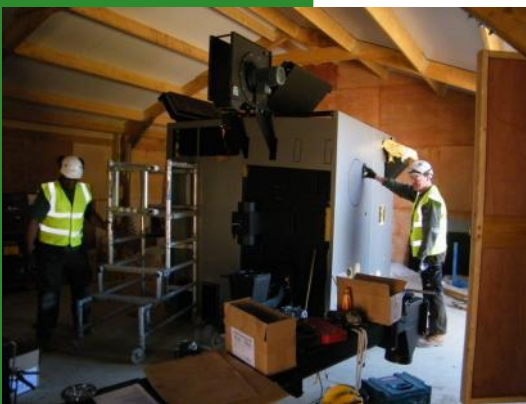
Below: Biomass boiler being fitted
