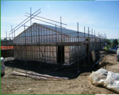
Above: Boiler room and workshops under construction
