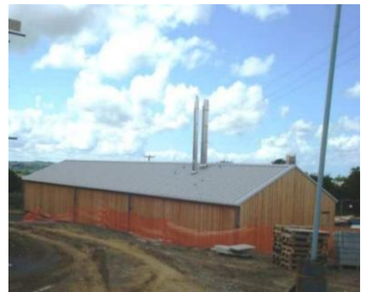
Above: The finished workshops and boiler house showing the raised chimneys.
